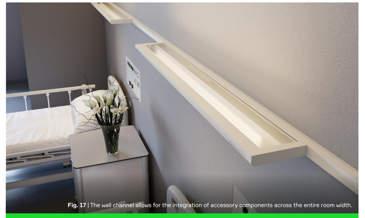
Fig. 17 | The wall channel allows for the integration of accessory components across the entire room width.
